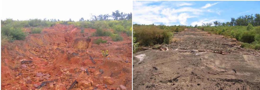
Figure 7: Eroded rehabilitation area (left) and the same area following erosion control works (right) in Western Australia.
